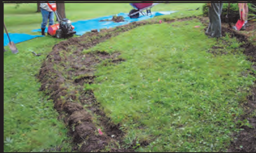
Build the berm with sod
